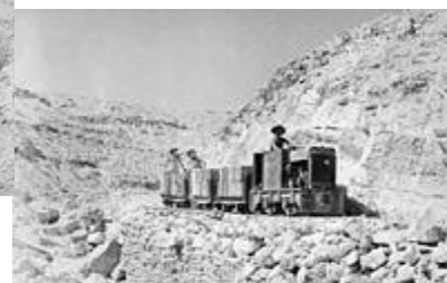
Narrow gauge train above a wadi at the eastern side of Tobruk harbour
