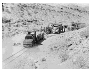
Loading the trains east of the harbour
