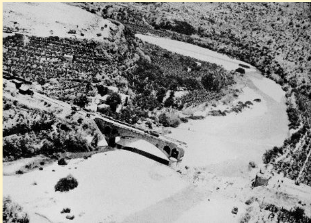
Broken bridge at the mouth of the Damour River
