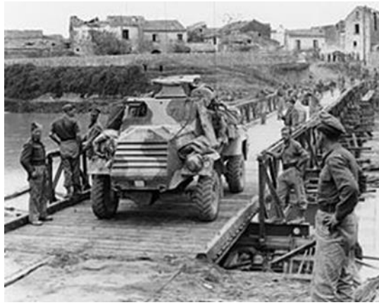
An Otter crossing a Bailey bridge over the Voltorno river at Grazzanise in Oct 1943
